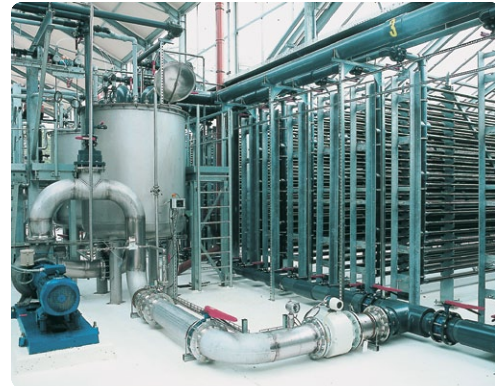
Figure 13: Photobioreactor for the production of green algae (picture: IGV GmbH)
